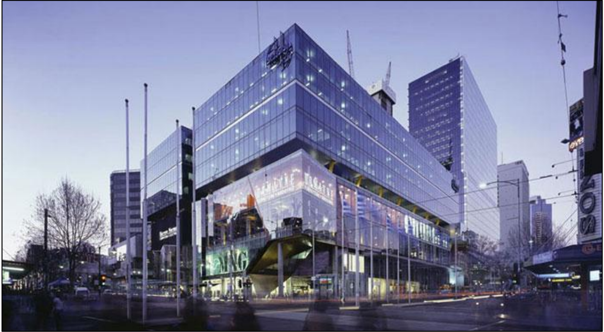
Figure 13 - External view of the QV Development
